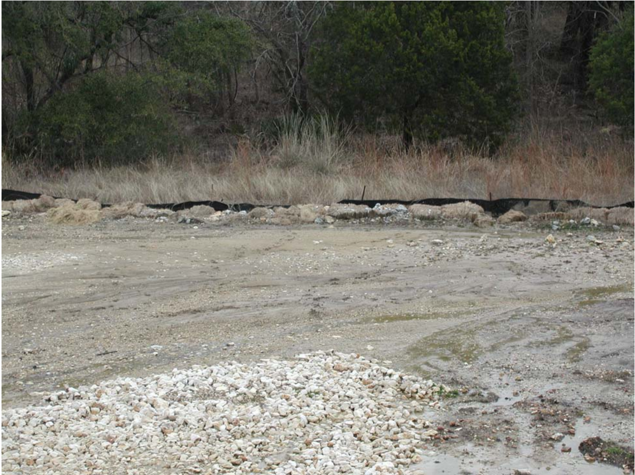
Failed silt fence.
