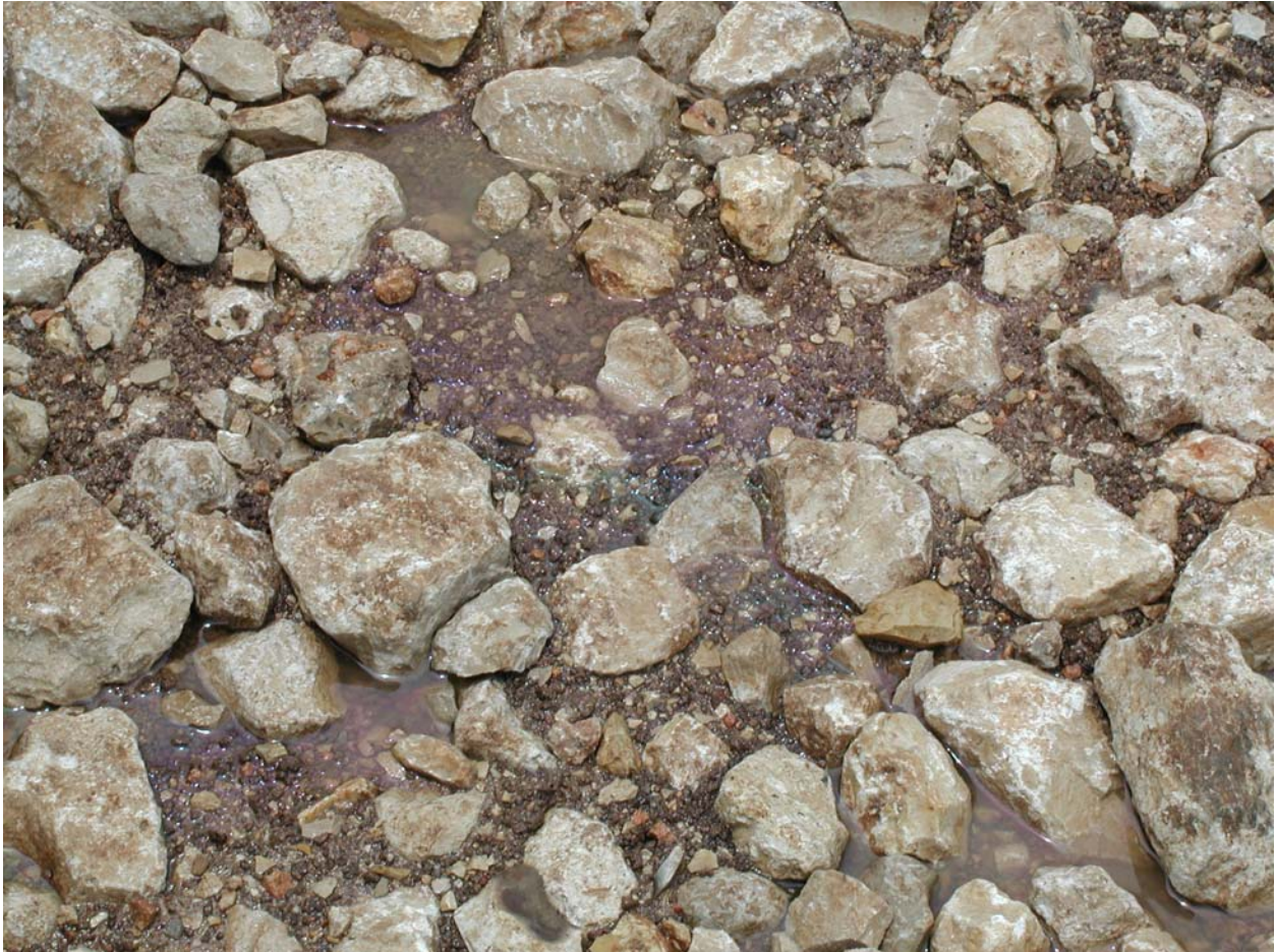
Leaked fuel on the stabilized construction entrance rock.
