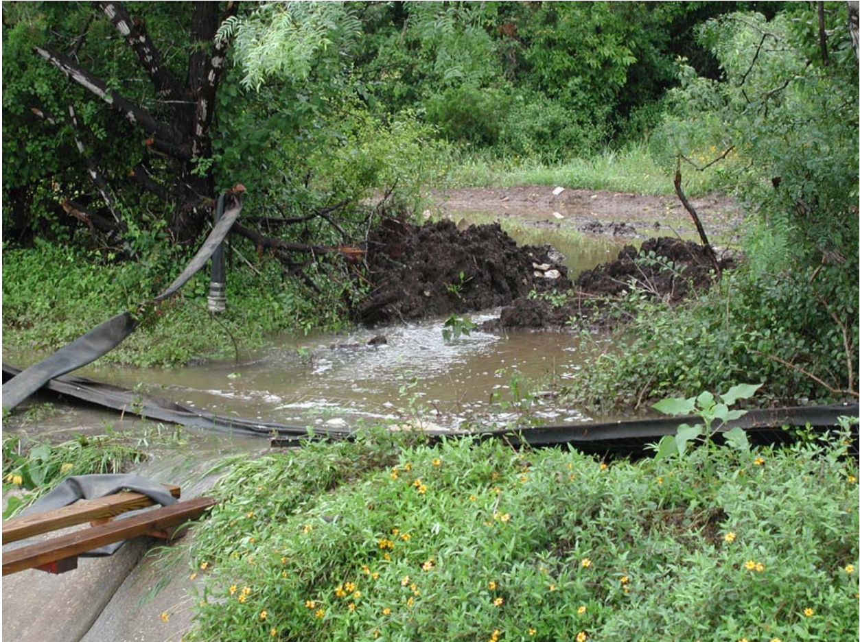
Silt fence failure following rain event.
