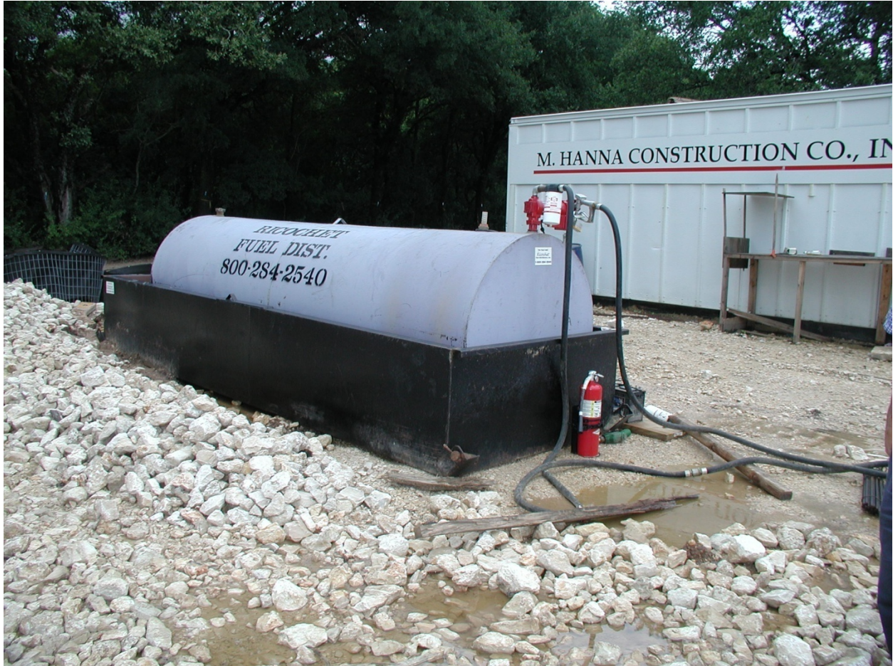
Leaking fuel storage system.
