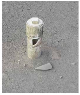
Broken cleanout pipe in sand filtration unit
