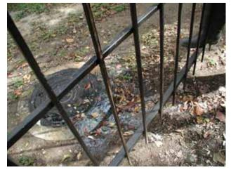
Raw sewage spilling from a sanitary sewer
